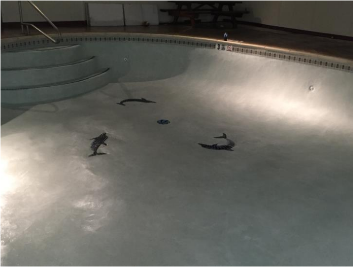
Finished and ready to fill
